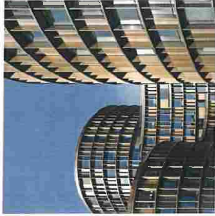
Axel Towers, Lundgaard Tranberg
