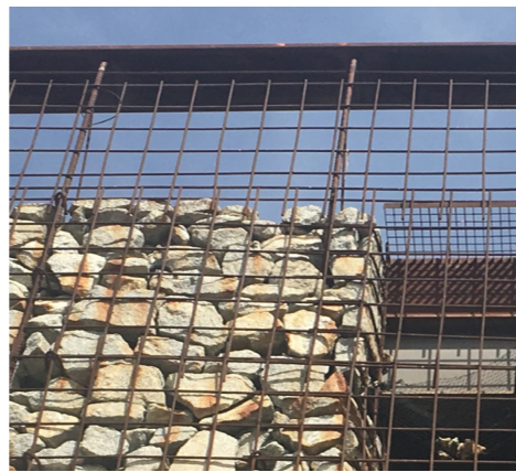
Gabion / Gabionmur
