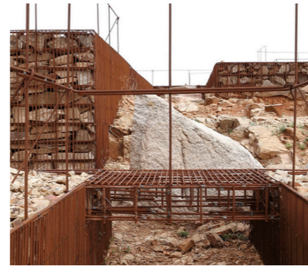
Gabion / Gabionmur
