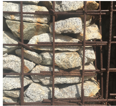
Gabion / Gabionmur
