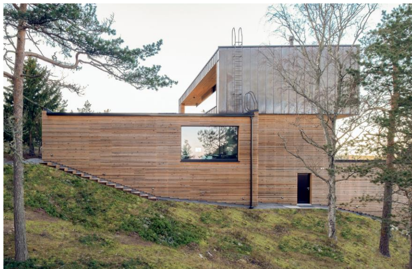
II. Fasad trapphus
