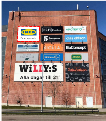
South facade towards the roundabout.
