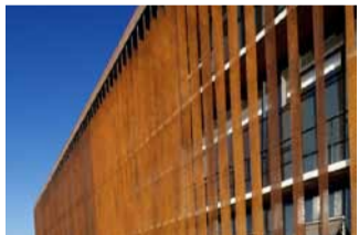
Ferreteria O'Higgins / GH+A
