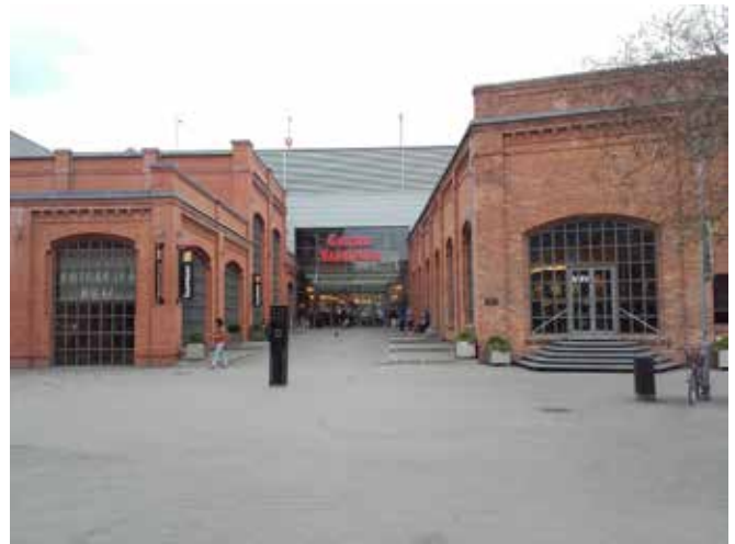
Site visit with architect Jaroslav Dokoupil
