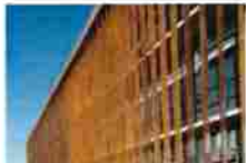
Ferreteria O'Higgins / GH+A
