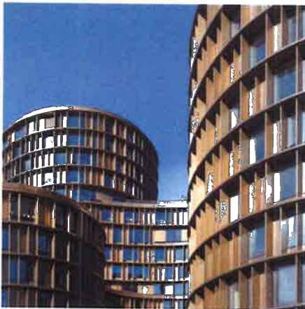
Axel Towers, Lundgaard Tranberg
