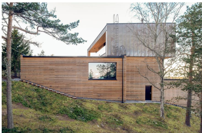
II. Fasad trapphus
