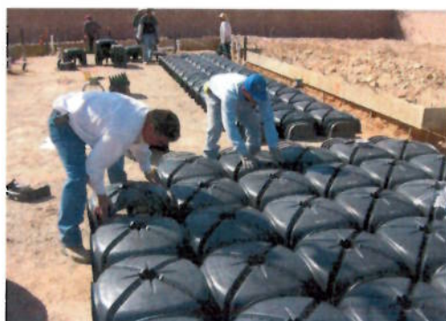
Figur 10a. Cupolex® former placeras ut under bottenplattan.
